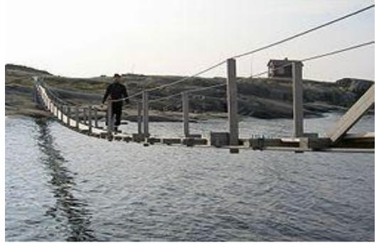
simple suspension bridge rare essentially thickened cables, and follow a catenary curve. A stressed ribbon bridge is a more sophisticated structure with the same catenary shape see [11]
