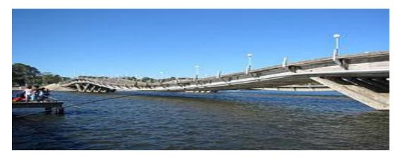
(Stressed ribbon bridges, like this one in Maldonado, Uruguay, also follow a catenary curve, with cables embedded in a rigid deck.)
